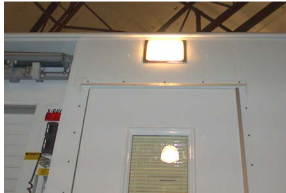
Figure 46: Staff Door Lighting
