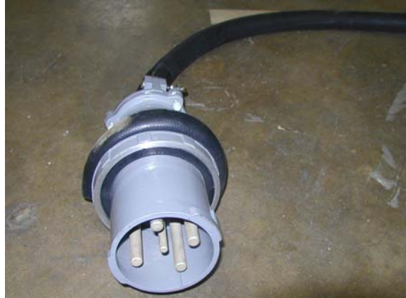
Figure 26: Shore Power Connection
