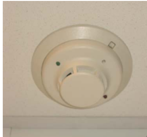
Figure 18: Smoke Detector
