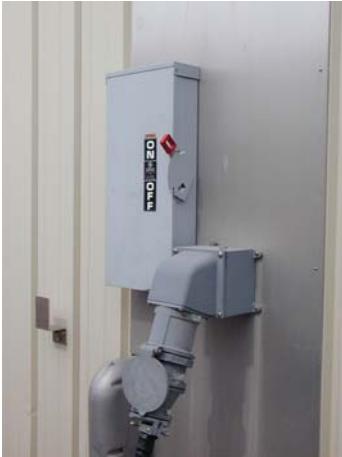
Figure 26: Shore Power Connection
