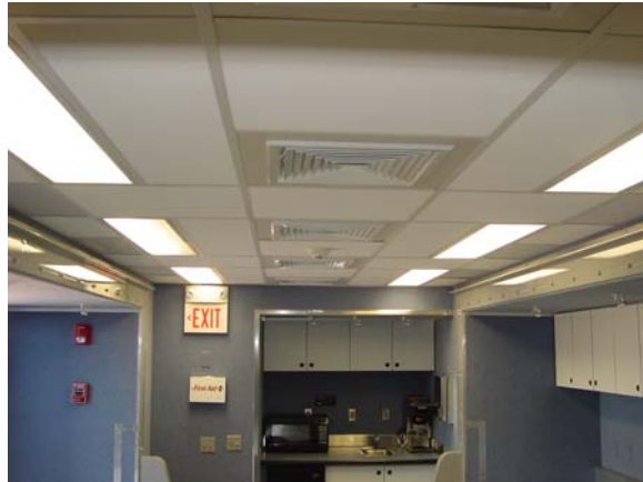
Figure 38: Command Room #3 Overall Lighting
