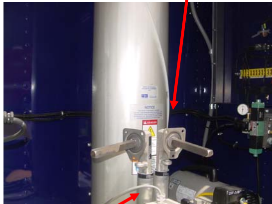
Figure 15: Expando Restraint Hardware
