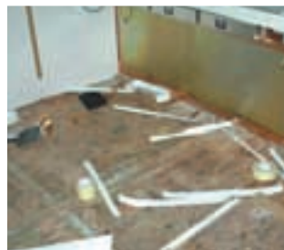
Removal of Damaged Areas
