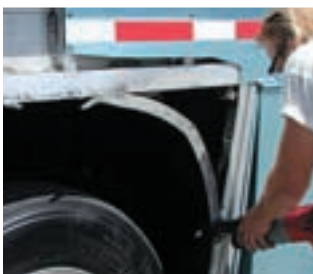
Removal of Damaged Areas
