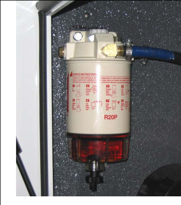
60KW Generator application
