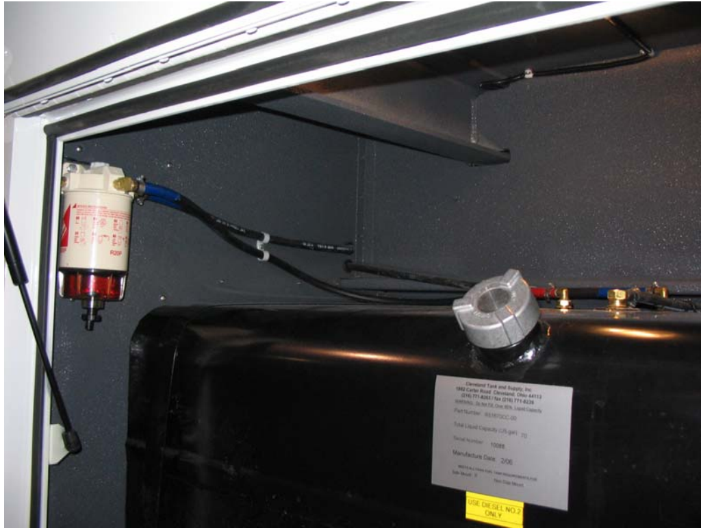
Figure 4. Lower Compartment After Installation
