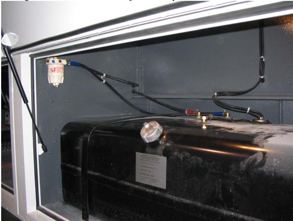
Figure 5. Lower Compartment After Installation
